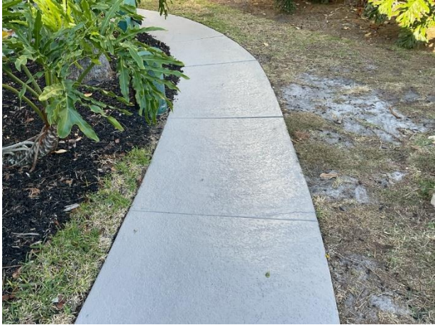
Concrete sidewalk with coating
