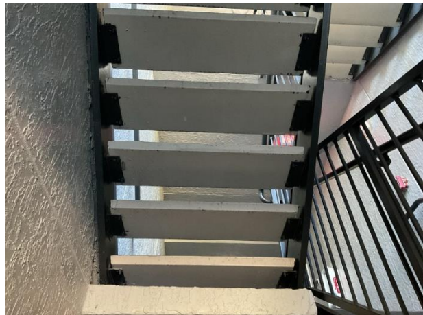
Metal staircase with concrete treads
