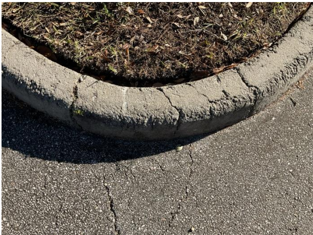
Concrete cracks
