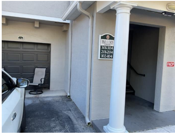
Aluminum gutters and downspouts
