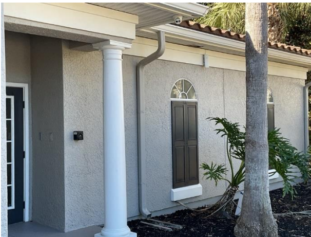
Aluminum gutters and downspouts
