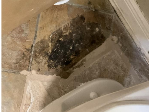
Pool rest room floor previous repair
