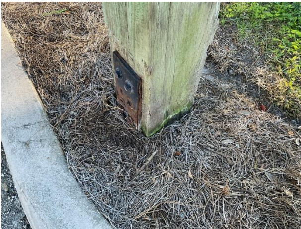
Pergola wood deterioration
