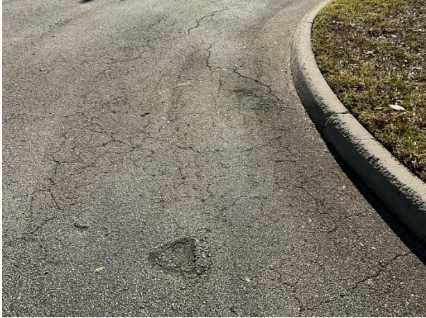
Pavement cracks
