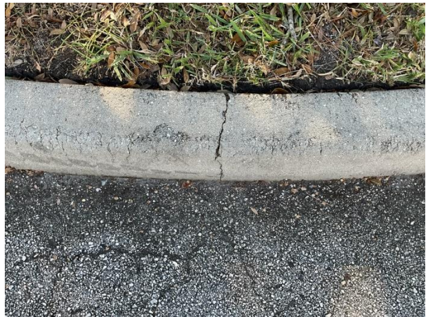
Concrete cracks
