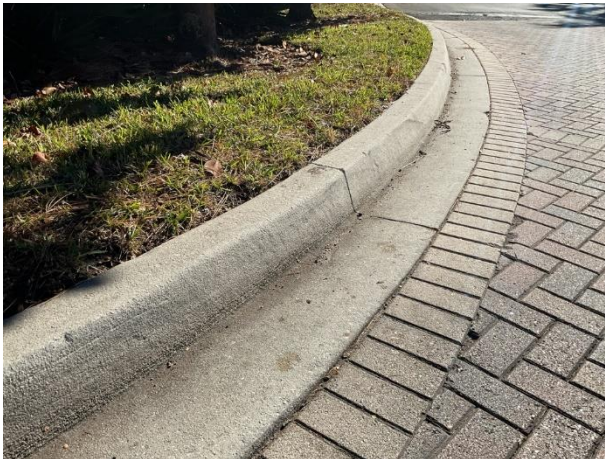
Concrete curb and gutter
