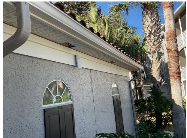
Aluminum gutters and downspouts
