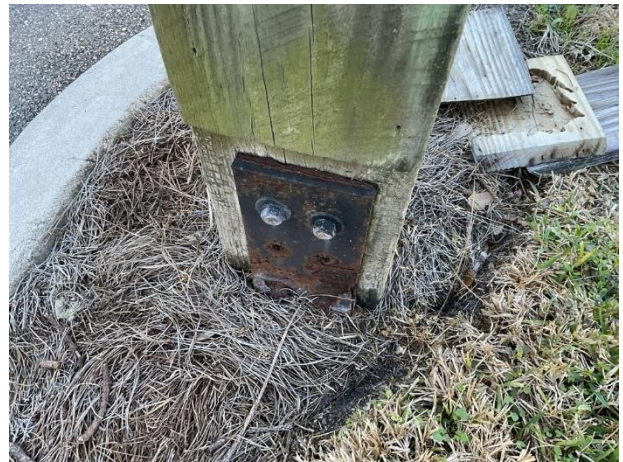
Pergola wood deterioration
