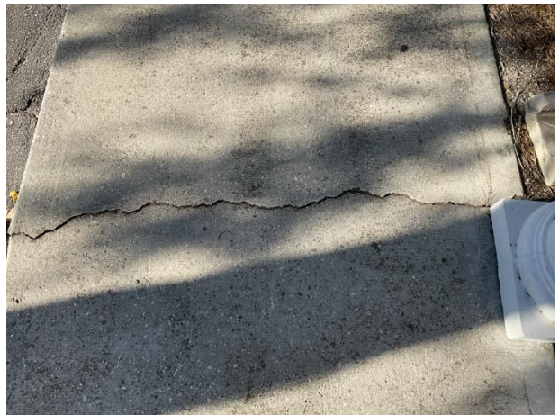
Sidewalk cracks
