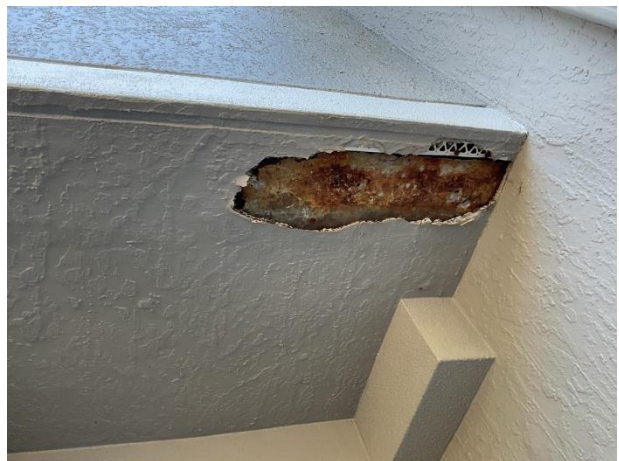
Evidence of water infiltration
