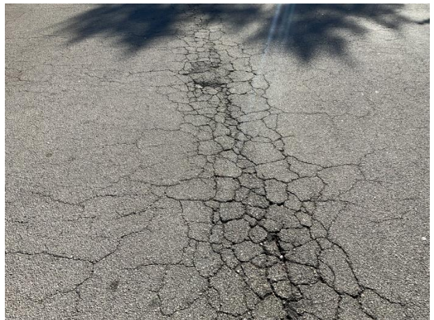
Pavement cracks
