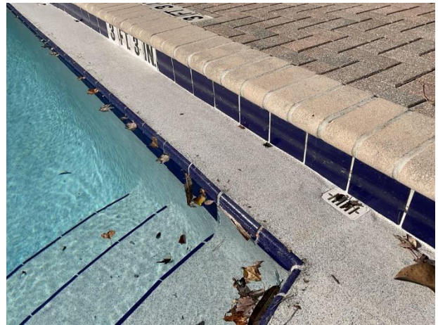
Pool plaster finish with tile perimeter
