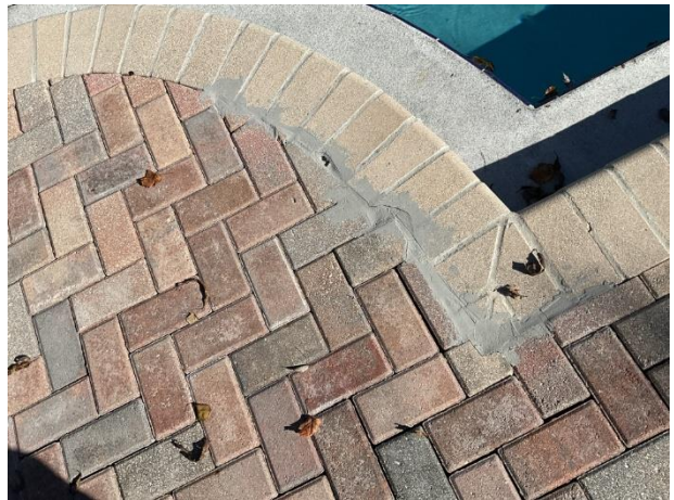
Paver pool deck previous repairs
