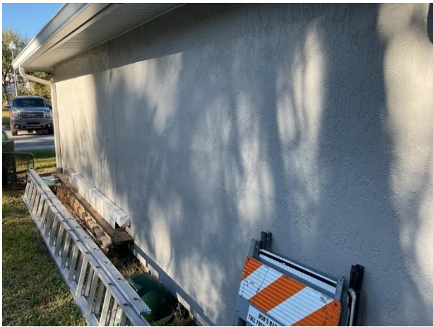
Stucco wall finishes at maintenance building
