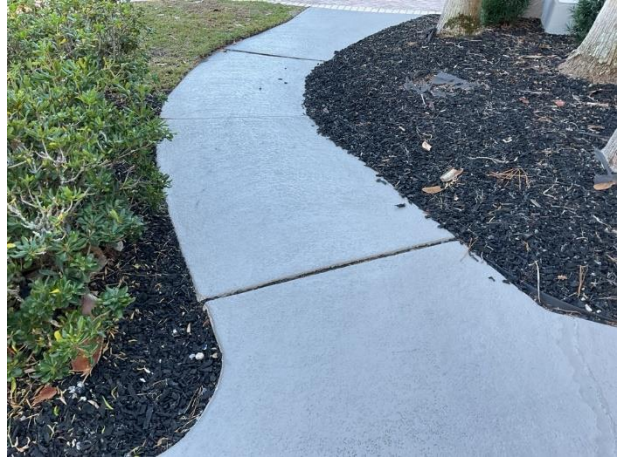
Concrete sidewalk with coating
