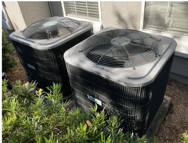
Split system condensing units
