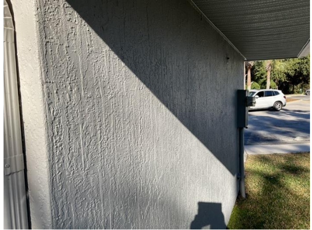
Stucco wall finishes at maintenance building
