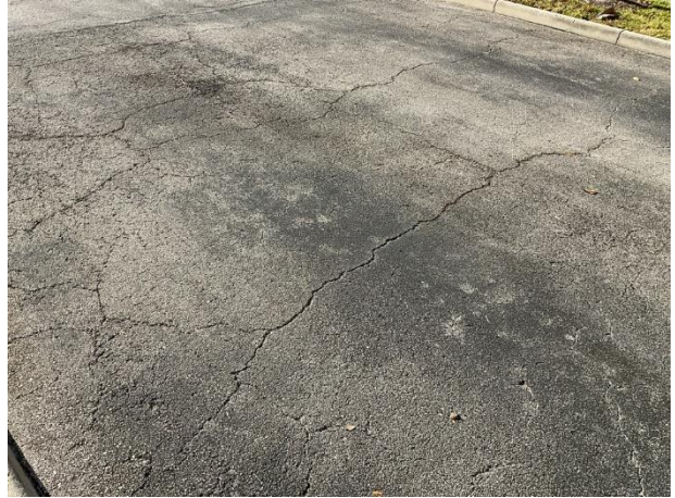
Pavement cracks
